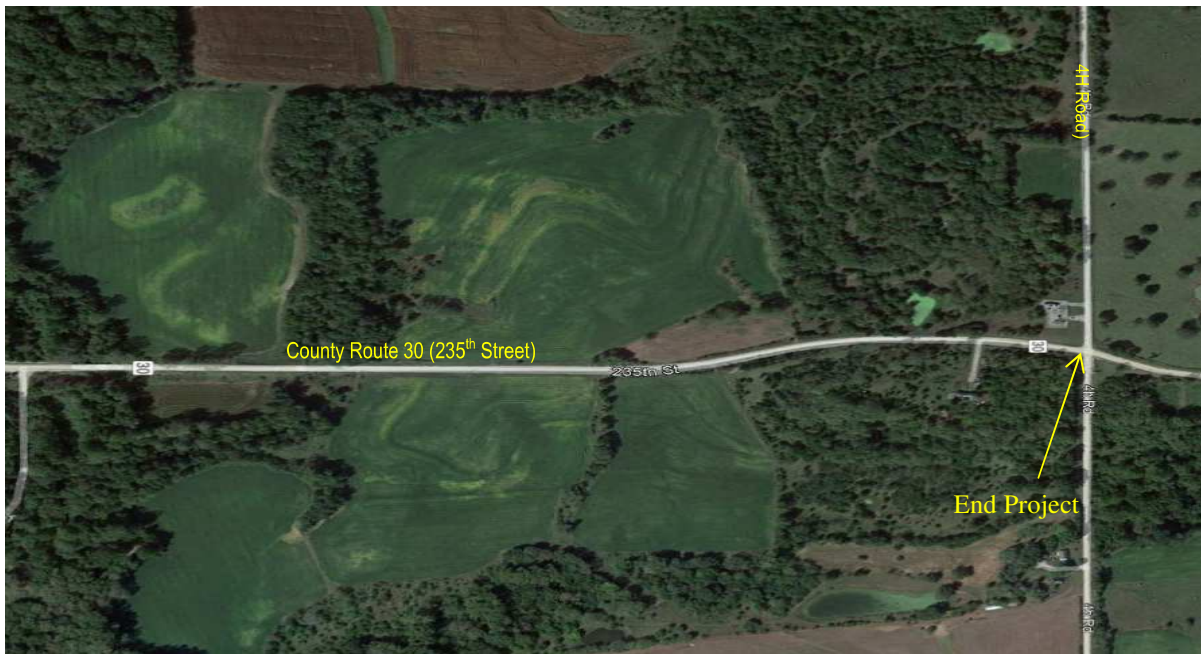
Figure No. 3 – Aerial view of final ½- mile section of road
